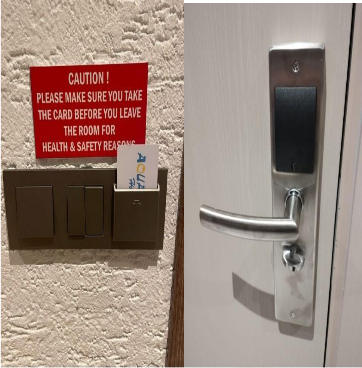
Our rooms automatically cut off energy when the energy card is removed, ensuring high energy savings.
